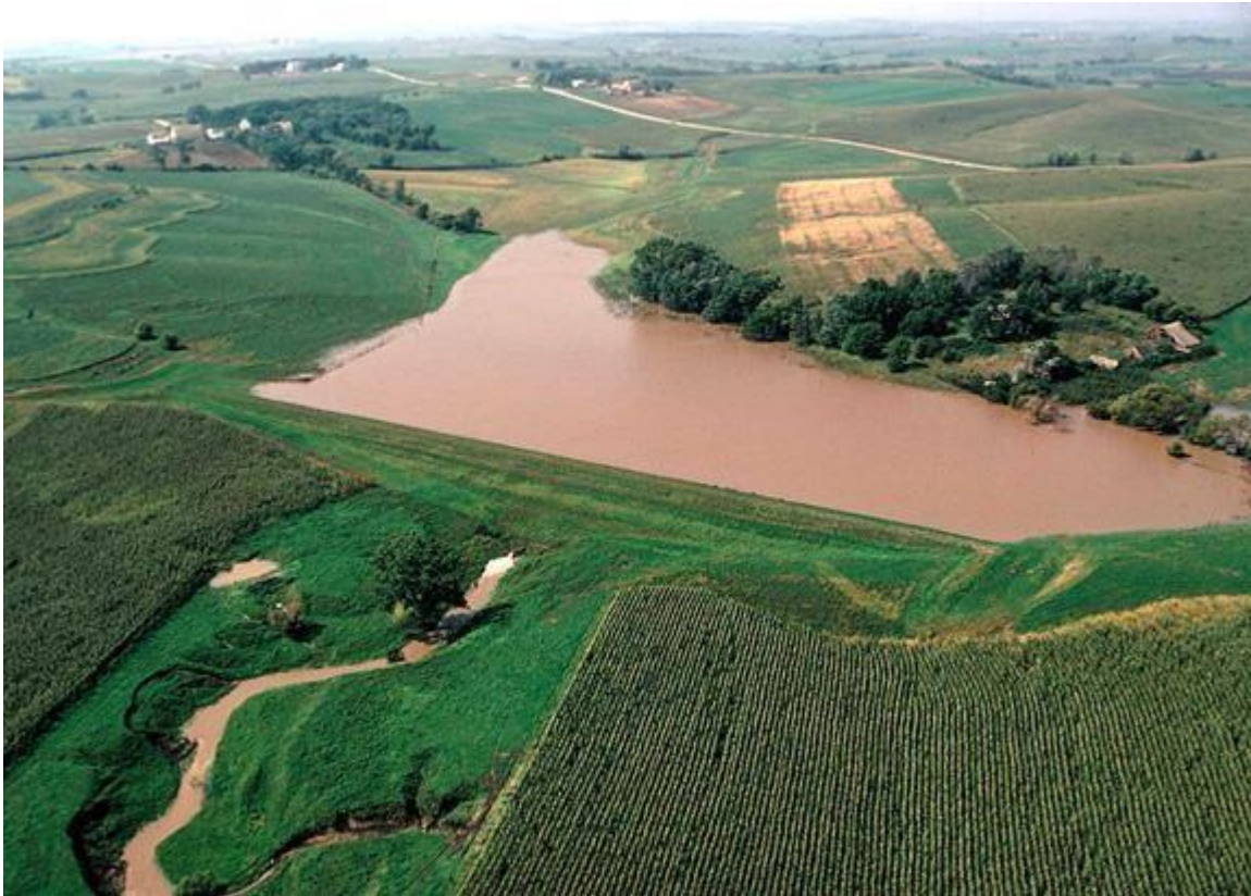
Figure 15. Small floodwater retarding structure in Iowa after severe rains.
