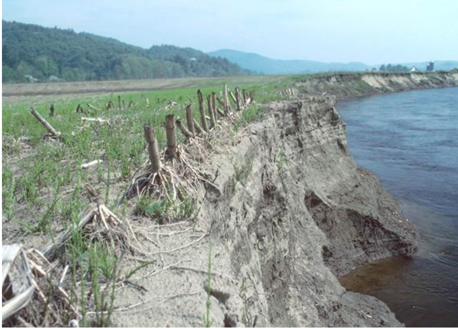
Figure 5. Streambank erosion occurring along major stream. Note missing rows of corn where the bank has eroded.
